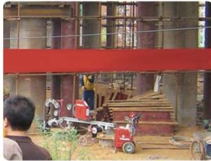
Synchronous lifting for replacement of bridge rubber bearings
