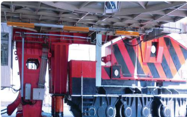
Long-term support for gantry crane maintenance
