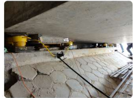
Synchronous lifting to replace rubber bearing for maintenance
