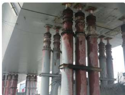
Synchronous lifting and docking of bridge slope adjustment
