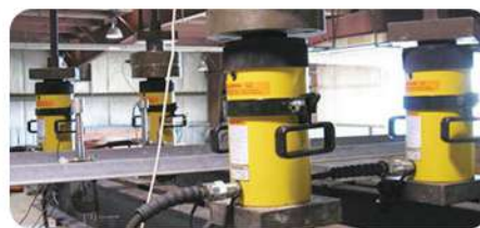
Synchronous lifting of steel structure assembly of gymnasium
