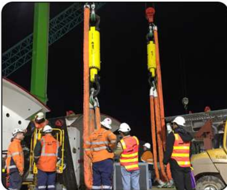
Precise positioning of segment hoisting for large shield machine
