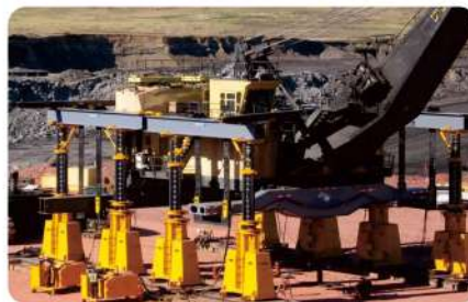
Lifting and Maintenance of Large Electric Shovel
