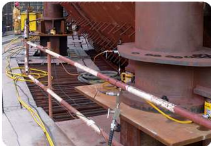
Synchronous lifting and positioning of nuclear island dome
