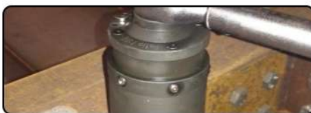
Steel structure bolt pre-tightening
