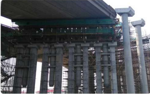
Long-term support for bridge elevation
