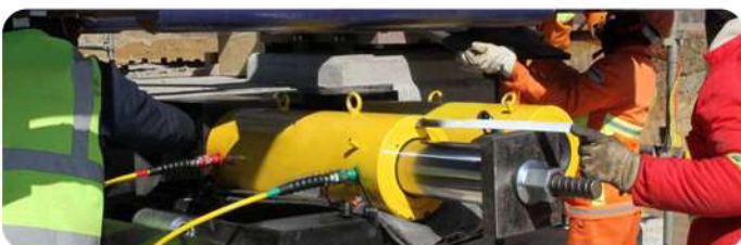
Bridge Construction Steel Structure Synchronous Traction
