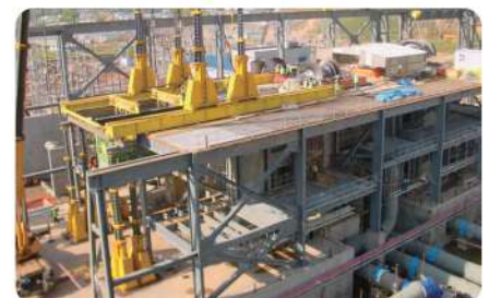
Lifting and Installation of Large Generator
