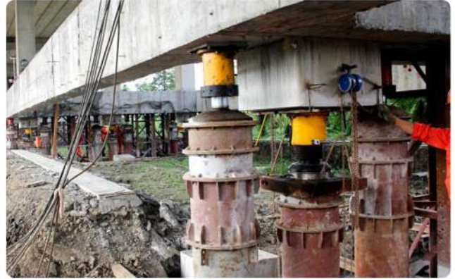
Synchronous lifting of large bridges as a whole
