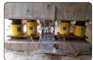
Alternate synchronous jacking of highway bridges
