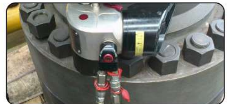
Chemical plant high pressure pipeline flange bolt pre-tightening
