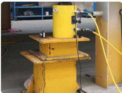
Synchronous lifting and weighing of large steel structures
