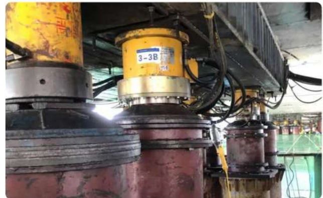
Long-term support for bridge elevation
