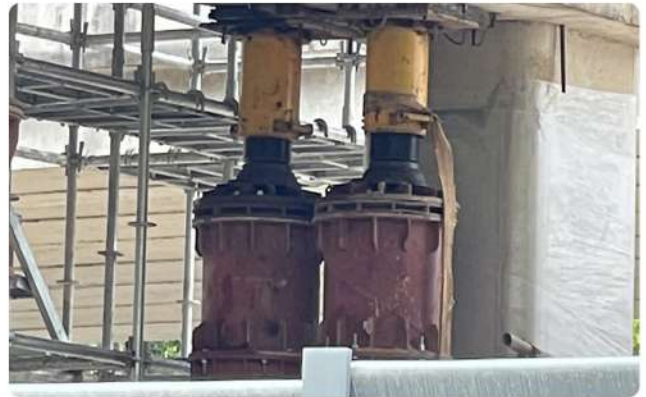
Synchronous lifting of bridge as a whole
