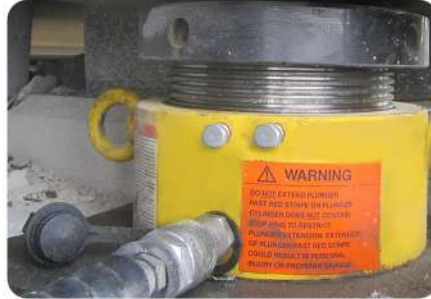
Synchronous lifting to replace the rubber bearing for bridge maintenance
