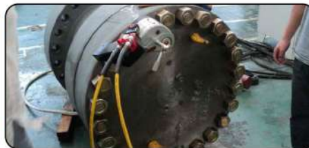
Steel mill high pressure pipeline flange bolt pre-tightening
