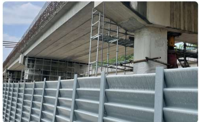
Synchronous lifting of bridge as a whole
