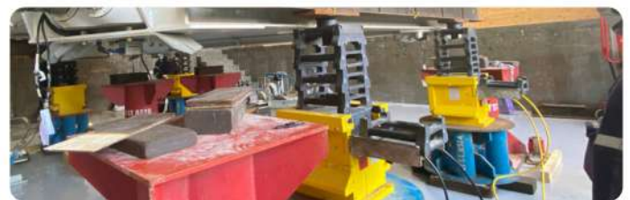
Synchronous lifting of large steel structures into place
