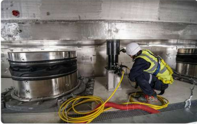
Synchronous lifting and installation of nuclear fusion Dewar base
