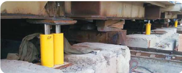
Synchronous lifting and replacement of steel plant blast furnace
