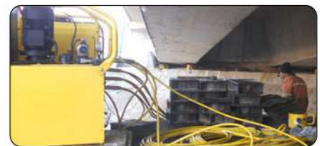
Synchronous lifting for bridge maintenance and replacing rubber bearings
