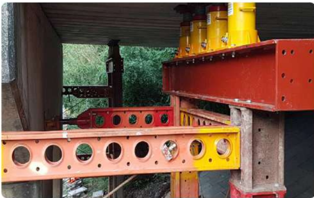
Synchronous lifting and replacing rubber bearings for bridge maintenance
