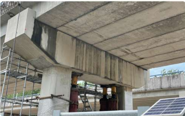
Synchronous lifting of bridge as a whole
