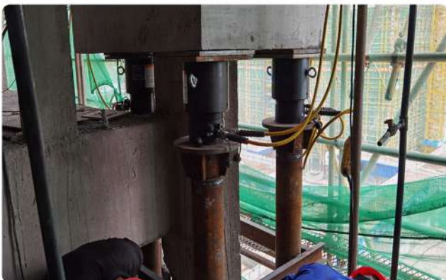
Building reinforcement concrete buttress underpinning
