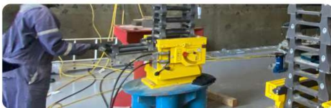
Synchronous lifting of large-scale equipment assembly into place
