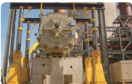
Lifting and Installation of Large Generator
