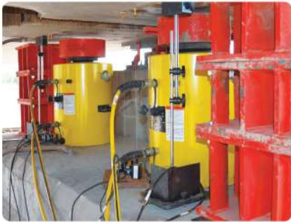
Synchronous lifting for High-speed railway bridge settlement remediation
