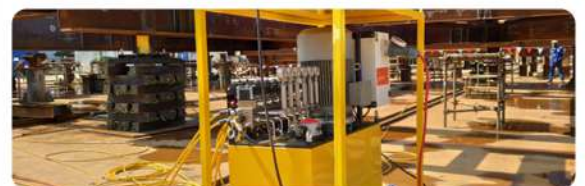
Synchronous lifting and weighing of drilling platform
