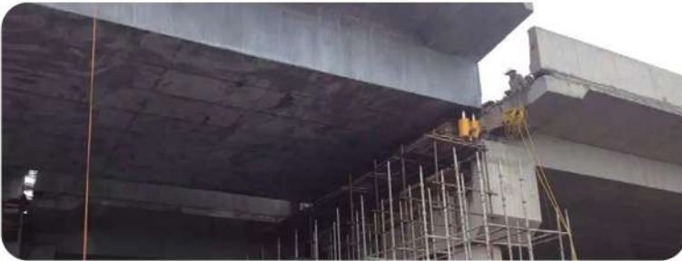
Synchronous lifting of lowering beam for bridge maintenance
