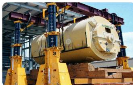
Lifting and Installation of Large Generator
