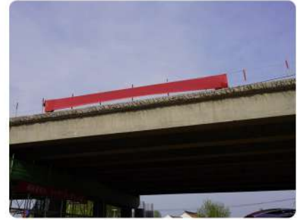
Synchronous lifting to replace rubber bearings
