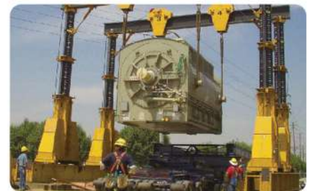
Lifting and Installation of Large Generator
