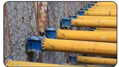
Synchronous intelligent support for foundation pits in subway construction
