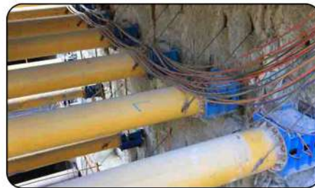
Synchronous intelligent support for foundation pits in subway construction
