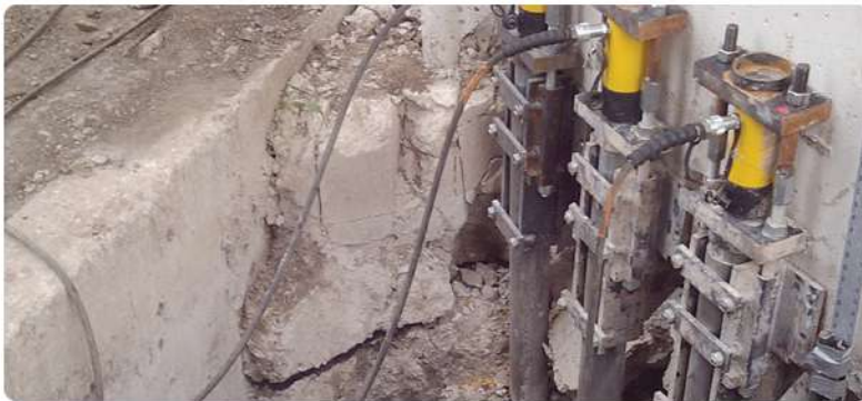
Synchronous lifting and correction of buildings
