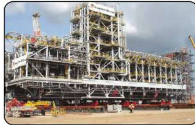
The liquefied petroleum gas regasification unit is pushed into place synchronously
