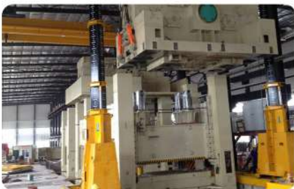
Lifting and Installation of Large Forging Press
