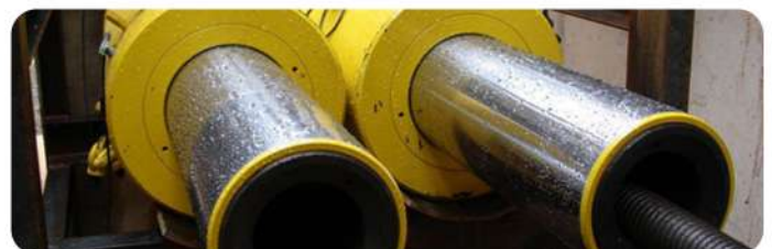
Synchronous traction of steel box girder
