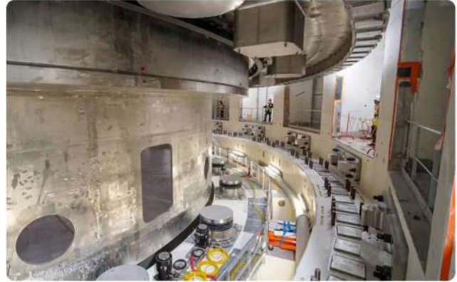
Synchronous lifting and installation of nuclear fusion Dewar base
