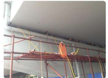
Synchronous lifting to replace rubber bearings for bridge maintenance
