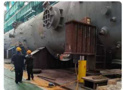
Synchronous lifting and moving of large pressure vessels
