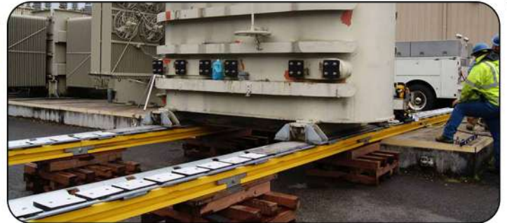
Transformer pushed into place
