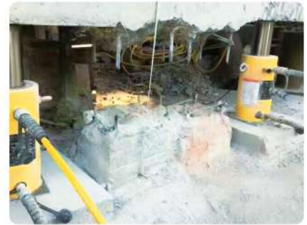
Synchronous house lifting, rectification and translation
