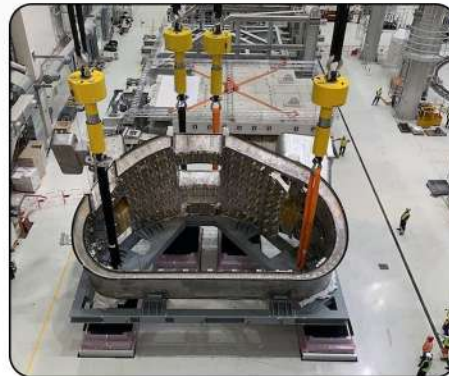
Precise positioning of nuclear power component hoisting
