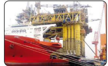
Synchronous push and loading of drilling platform
