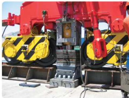
Synchronous lifting for 500T port floating crane maintenance
