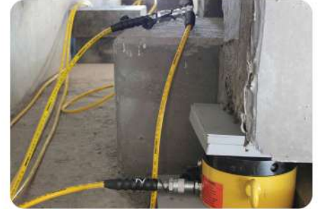
Synchronous lifting to replace the rubber bearing for bridge maintenance
