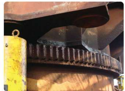
Synchronous lifting for large electric shovel maintenance
