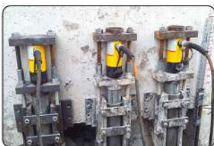
Building Rectification and Jacking
