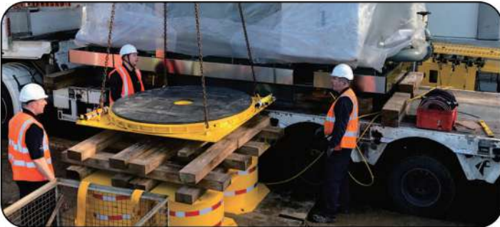
Transformer pushed into place
