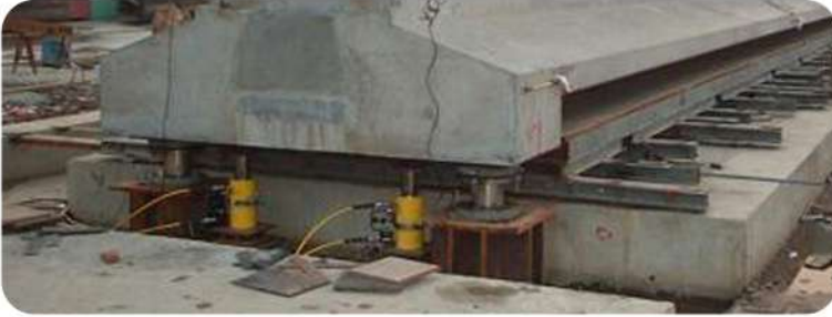
Synchronous lifting and fine adjustment of maglev track construction
