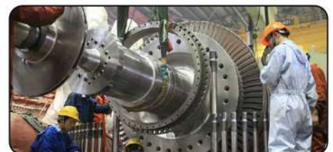
Dismantling of maintenance bolts for steam turbines in thermal power plants
