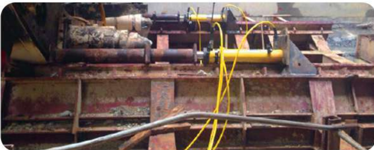
Lifting and installation of shield machine
