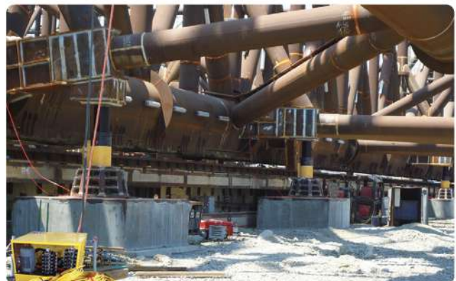
Synchronous lifting and installation of large steel structure
