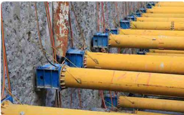
Axial load support for subway construction
