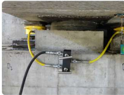
Synchronous lifting to replace rubber bearings for bridge maintenance
