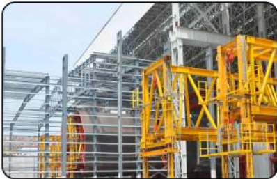
Undersea tunnel construction caisson synchronously pushed into place
