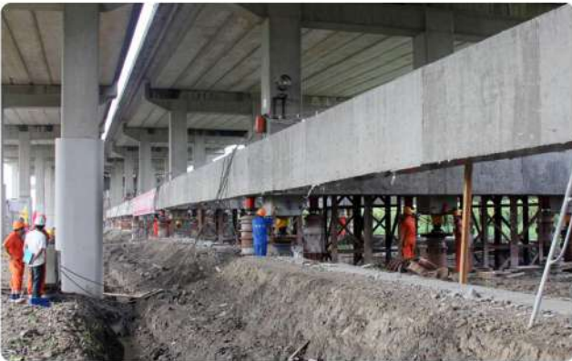
Synchronous lifting of large bridges as a whole
